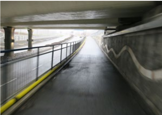
Tunnel under Södervägens bro
